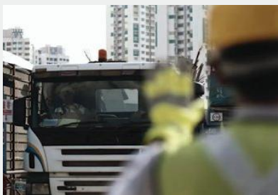
Trained banksmen directing/manoeuvring vehicle.
